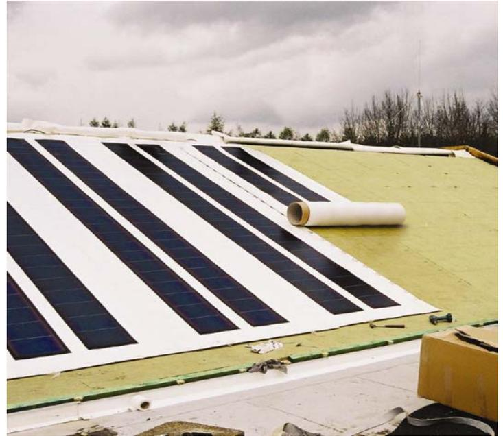
**FIG 2:** Roofing membrane being laid down at another project
